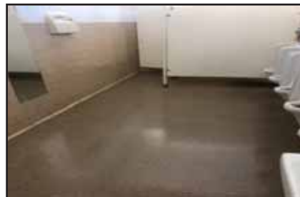
The mens restroom after
